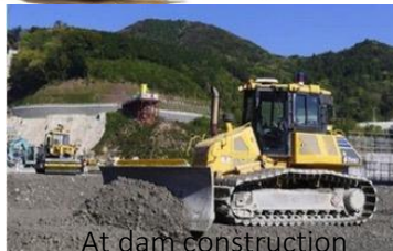
At dam construction
